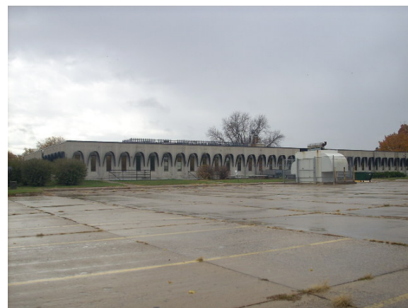
4. View of Iowa Telecom site facing southwest
